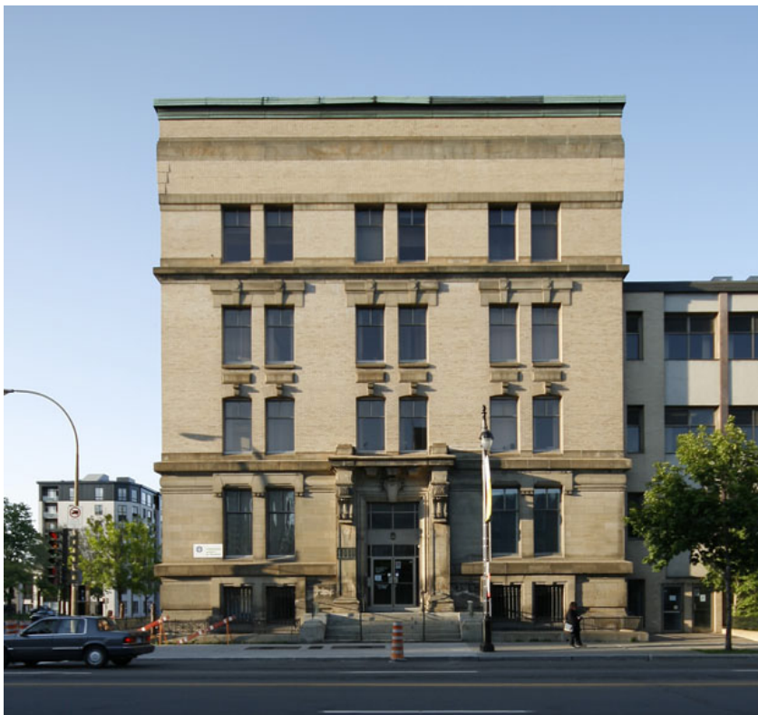
École du Meuble's façade, at 1097, Berri Street, after architectural modifications. Photo: Alexis Hamel, January 2008.
