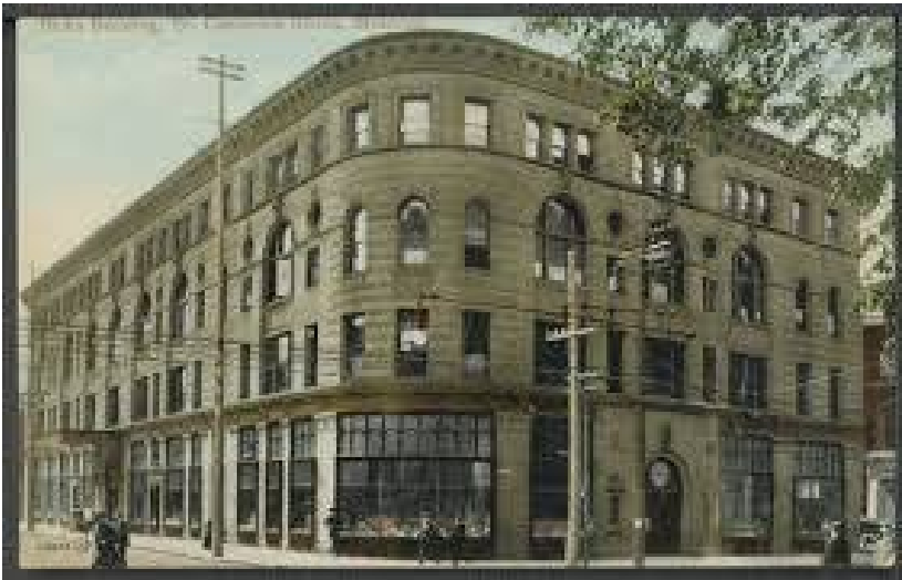
Maison Birks, Sainte-Catherine Street. Architect: Edward Maxwell. Photo: BANQ.
